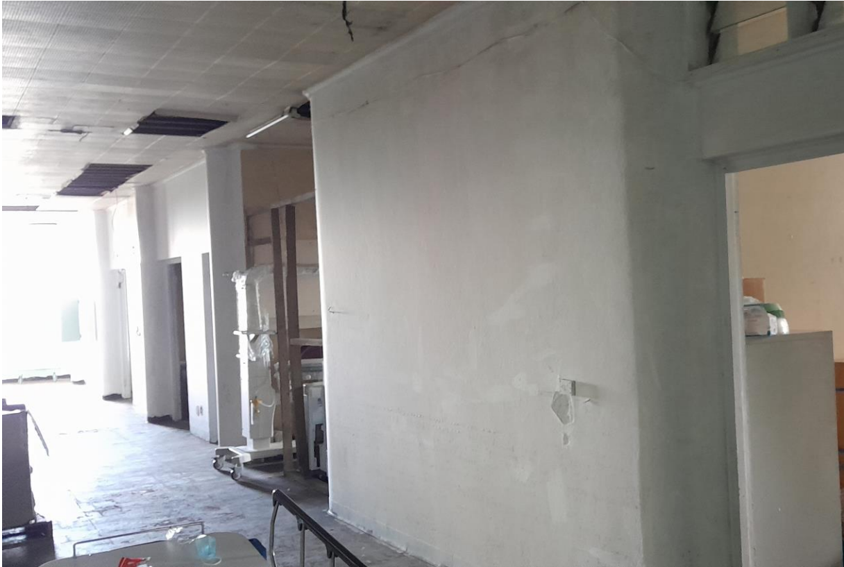
Figure 12: Old OT hallway post paint work, March 2023
